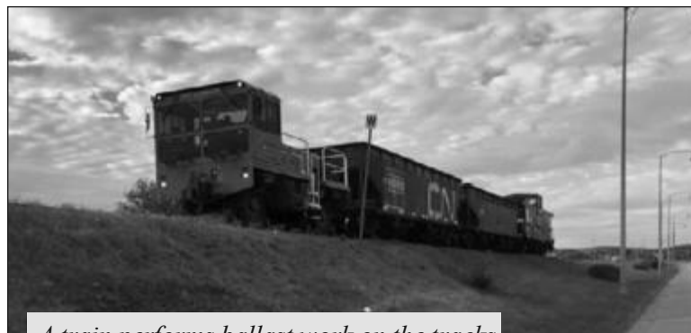
A train performs ballast work on the tracks in the Port-Daniel-Gascons area.
